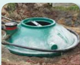
IPC access lid during installation
